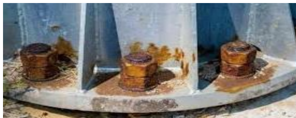
Figure 3 : Corrosion caverneuse
