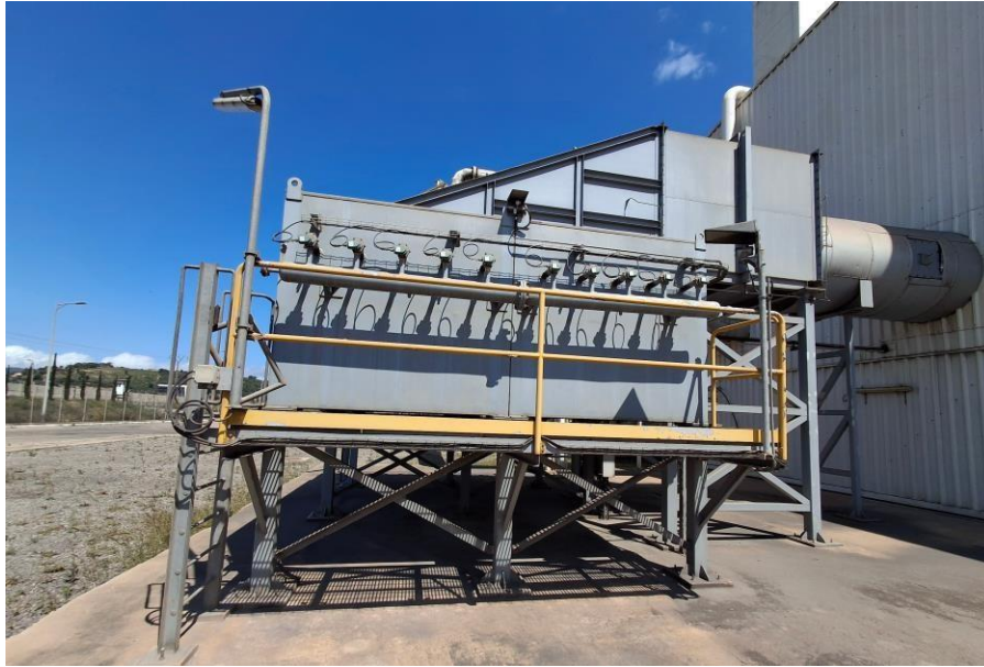
Appendix D.9: Real picture of air filter
