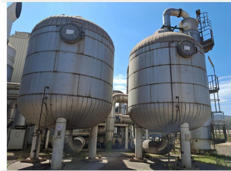
Appendix D.1: Real picture of the Molseive in the ASU
