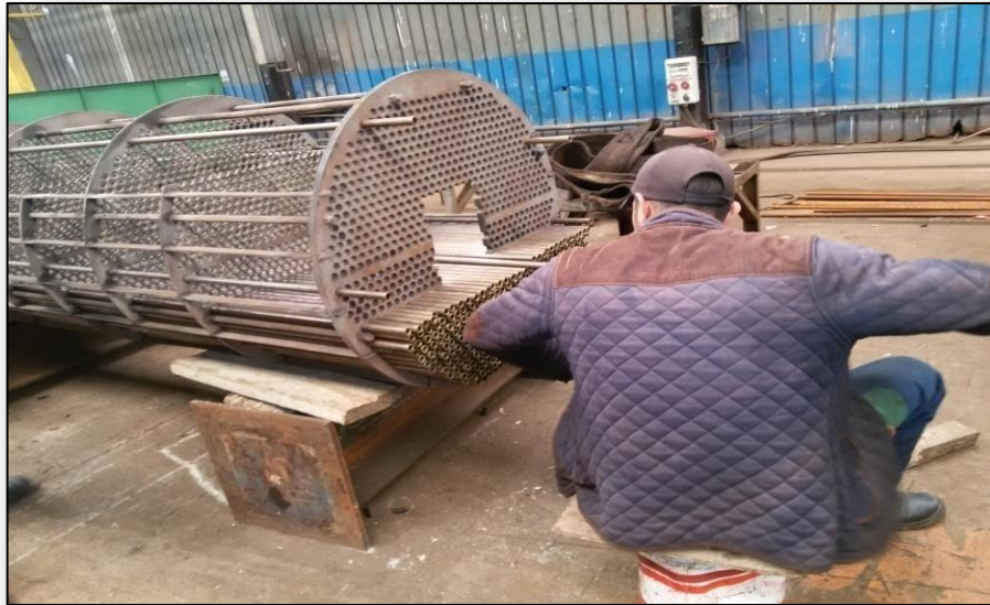
Figure V.2: retubage totale en cupronickel
