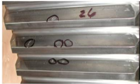
Figure I.5 Pitting ou piqûres
